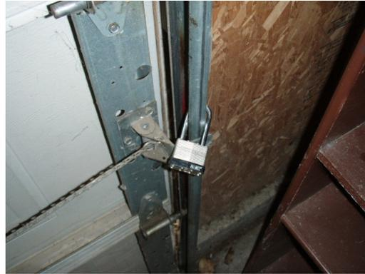
A pad lock in the garage door track can cause the door to fall off the tracks
