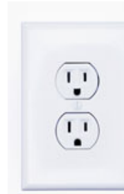
An unprotected outlet. How can you know which is which?
