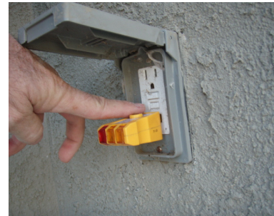
This GFCI failed to reset
